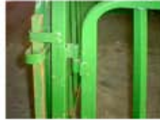
Handi-Klasp Style gate and pin assembly detail
